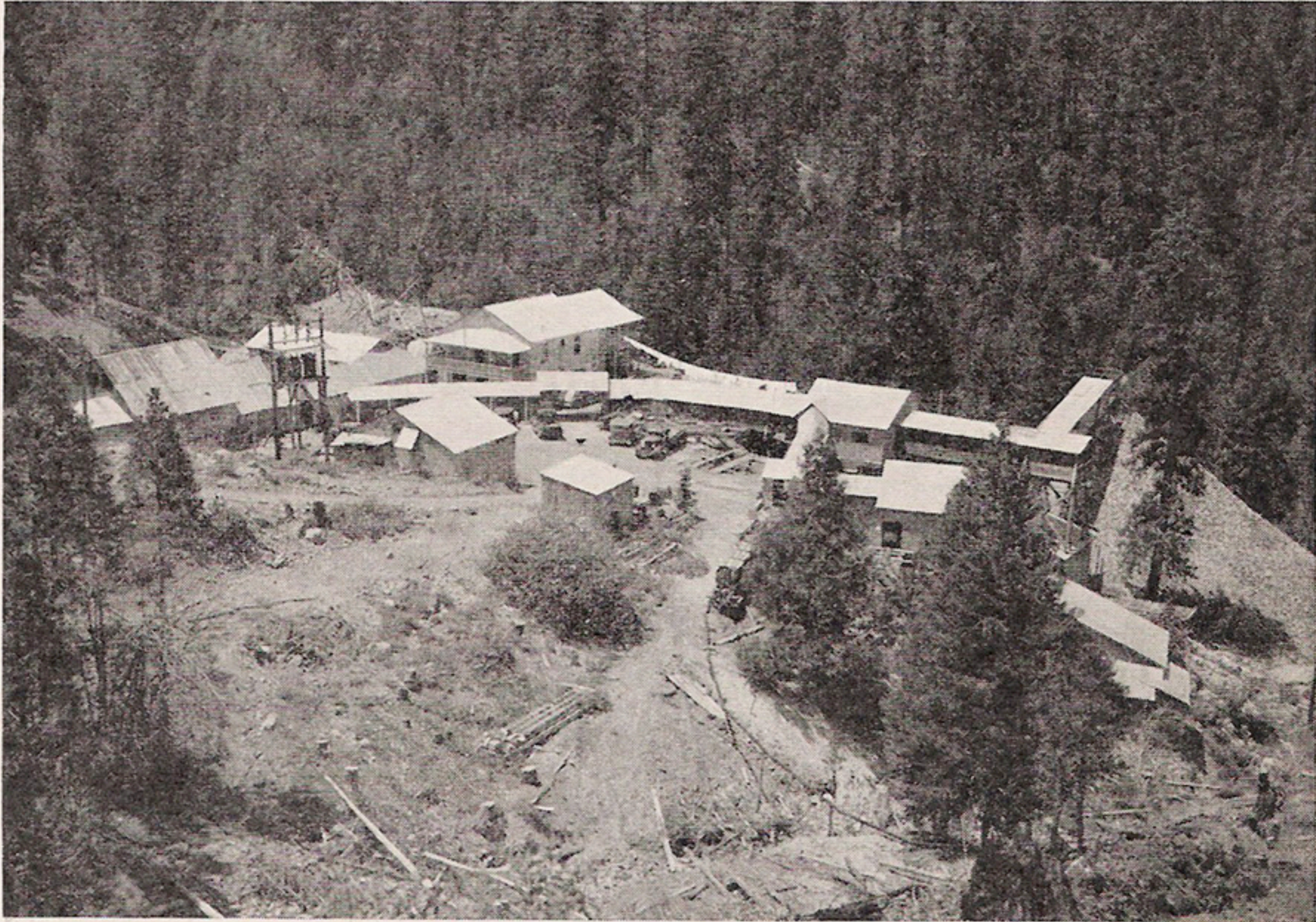
FIG. 11. Ruby Mine, surface plant
